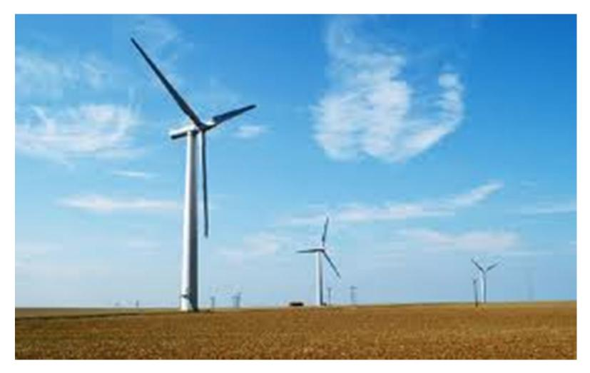
The wind blows the propellor round, which turns a generator to produce electricity.
